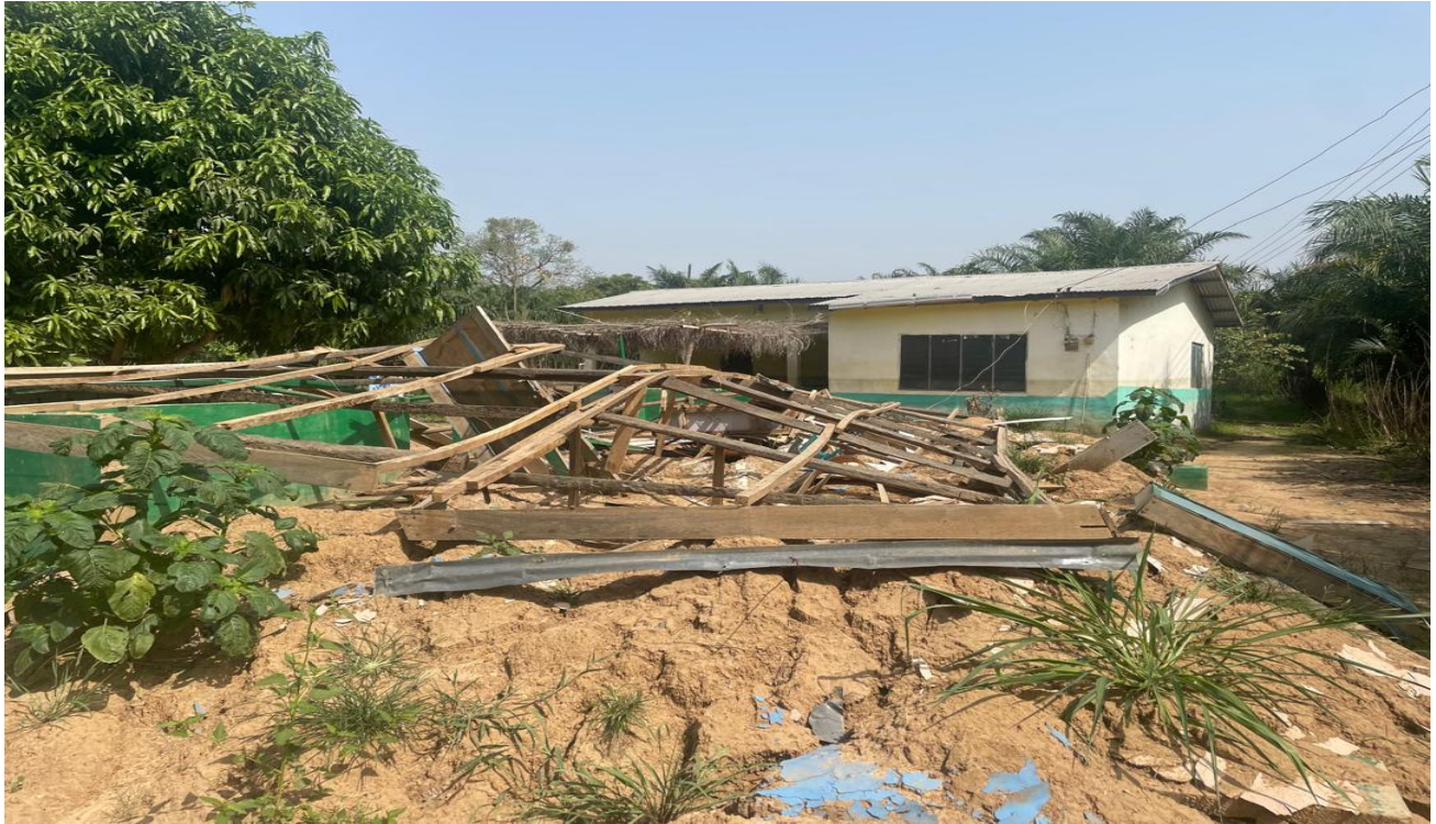
Figure 9 Damaged mud house of a victim (Source: Field Visit)
