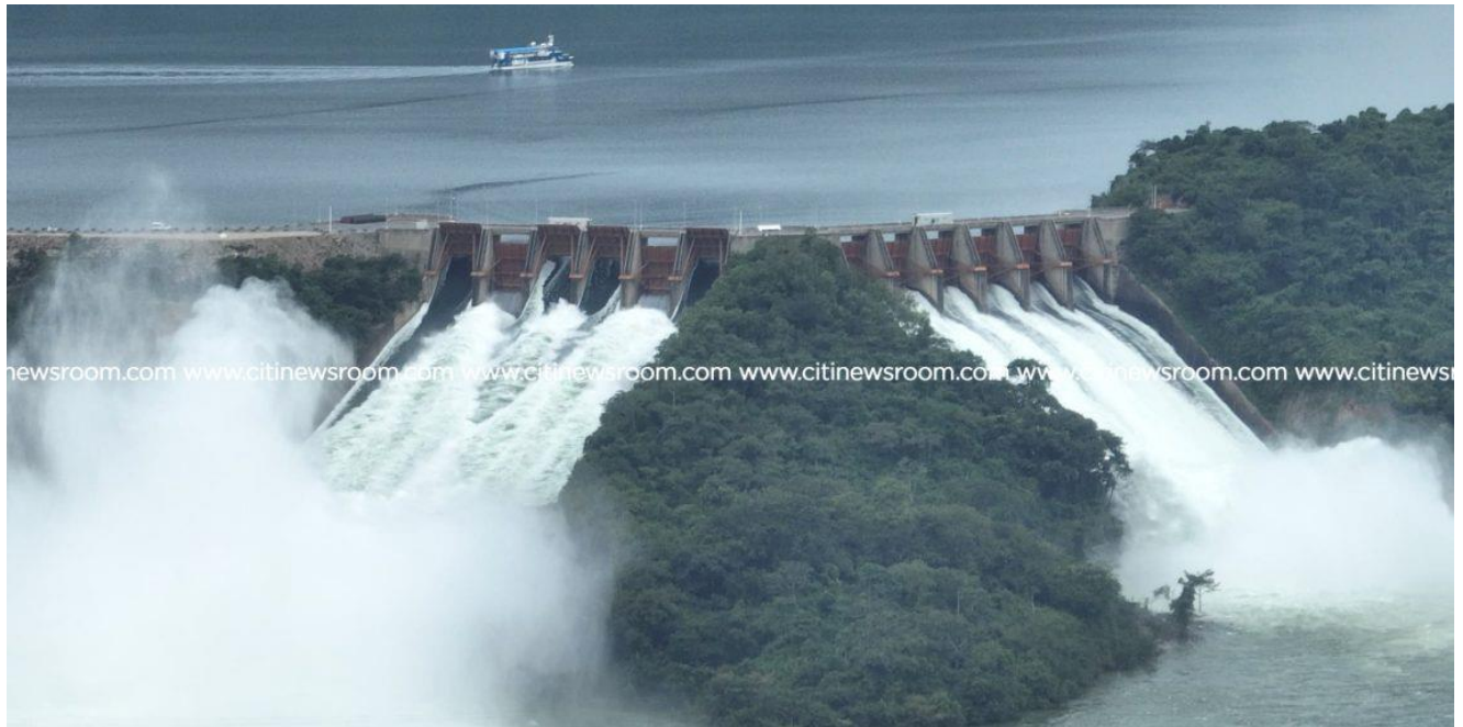
Figure 6 Akosombo Dam during the spillage (Source: Citinewsroom)
